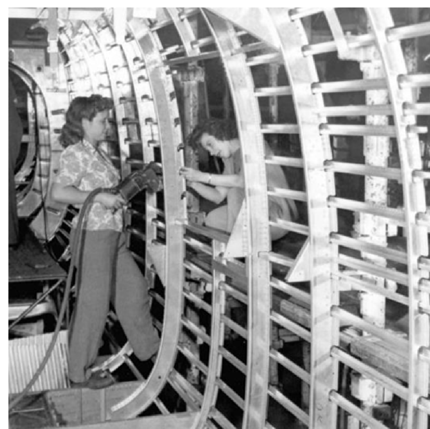
Women Assembling an Airframe, One with a Rivet Gun, Courtesy of San Diego Air and Space Museum.
